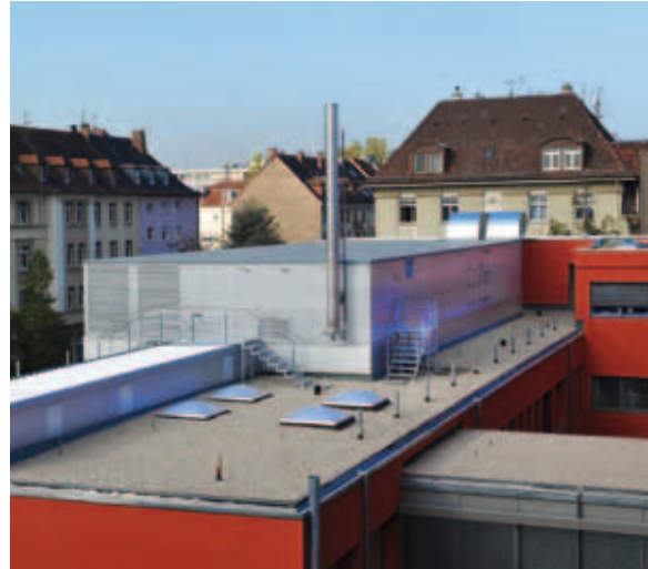
Roof control centre
