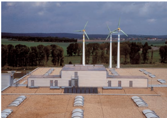
rooftop control system
