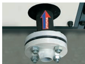
flange and pipe feed-through
