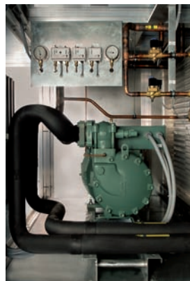
half hermetical screw compressor
